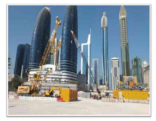
**PROJECT ABSTRACT:** This project involves the planning and execution of essential enabling works for DIFC Mixed Use Luxury Development on Plot No. 05 at Dubai, UAE. These works encompass shoring works, construction of preliminary test pile and bulk excavation.
